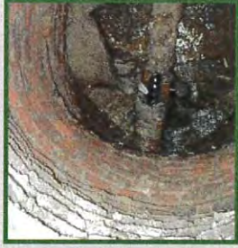
Broken sanitary sewer
