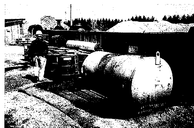
Secondary containment filled with stormwater.
