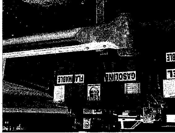
Leaking AST, in need of paint.
