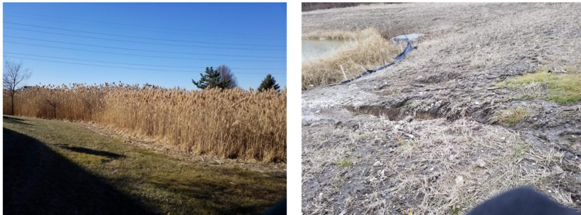
Figure 2-5 Basin Maintenance Vegetation Examples (Left) basin TY-03S10E28NWNE-3 is overgrown with phragmites. (Right) Vegetation in new basin FR-04S10E32NENE-1 has failed to establish, resulting in erosion and sedimentationFR-04S10E32NENE-1
